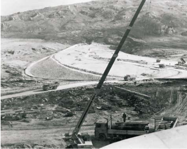
Fig. 38. The left abutment of the CASTELLO embankment dam near Agrigento (Sicily) rests on a large, stabilized landslide
