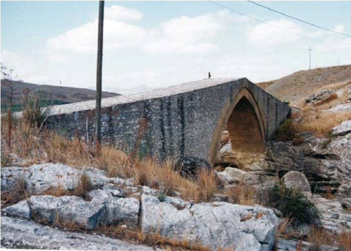
Fig. 60. The Calatrasi Bridge near the Rocks of Maranfusa in Sicily (photo by C. Gambino, 2002)
