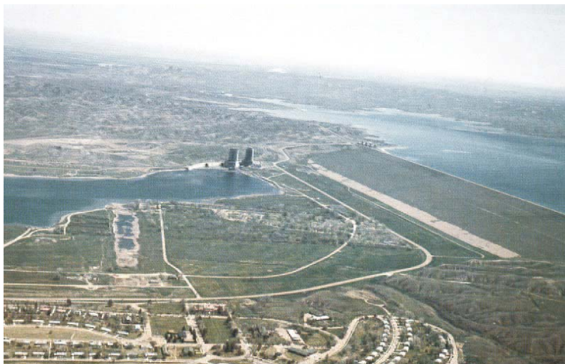
Fig. 92. The FORT PECK dam, USA, in service after the reconstruction of the right abutment [136]
