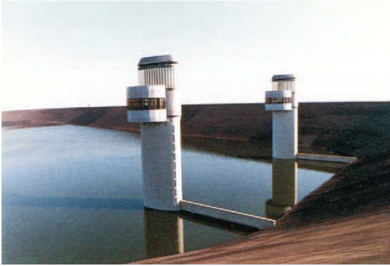
Fig. 70. The upper reservoir of the ANAPO pumped storage hydroelectric plant with its intake towers
