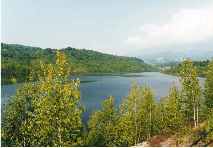
Fig. 65. The MONGRANDO reservoir on the Ingagna River near Vercelli, Italy, from the crest of the concrete section of the dam (1998)
