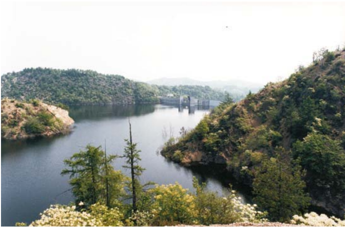
Fig. 66. The RAVASANELLA reservoir near Vercelli, Italy, from upstream (1998)
