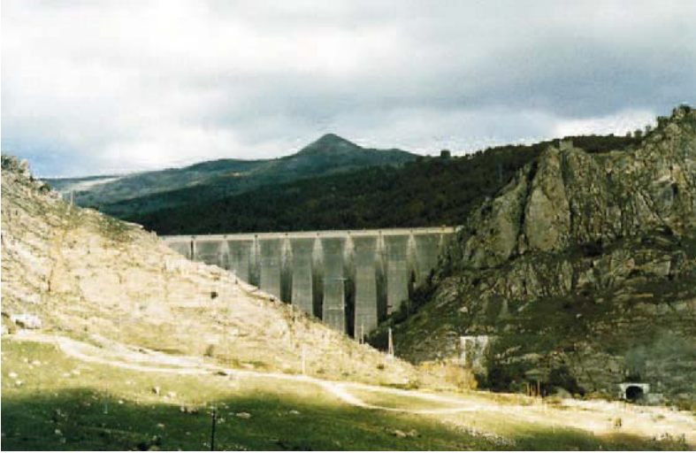
Fig. 8. The ANCIPA near Enna, Italy, is a gravity dam with hollow buttresses [64]
