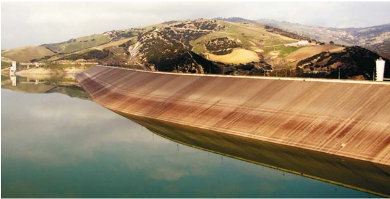
Fig. 7. The MONTE COTUGNO embankment dam on the Sinni River near Potenza, Italy [17]
