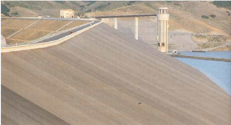
Fig. 84. The MONTE COTUGNO embankment dam on the Sinni River near Potenza, Italy [46]
