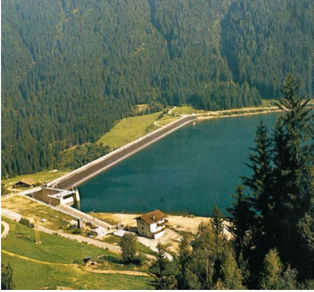
Fig. 36. The ZOCCOLO dam and reservoir from the left bank with the spillway and the guardhouse in the foreground [63]
