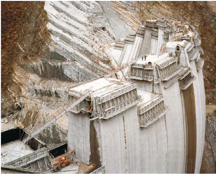
Fig. 112. The RIDRACOLI double curvature arch dam ( H = 100\text{ m} ) on the Bidente River in Romagna, under construction (L'Acquedotto della Romagna, 1991)
