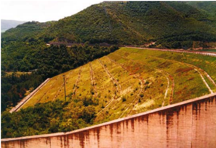
Fig. 63. The OCCHITO embankment dam on the Fortore River today
