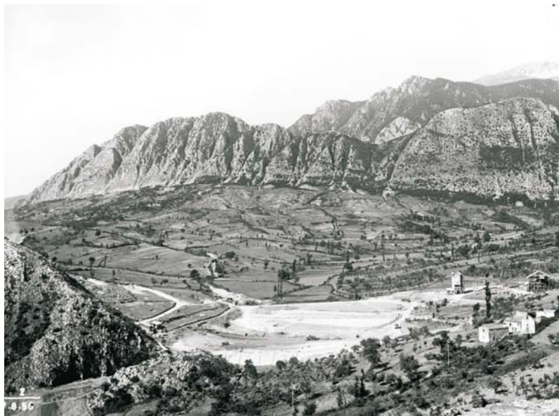
Fig. 76. The CASTELSANVINCENTO embankment dam near Isernia, Italy, under construction in 1956; the Mainarde chain of mountains rises in the background (photo by G. Chiolini)
