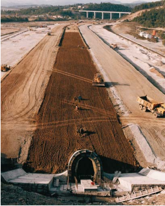
Fig. 89. The BILANCINO dam on the Sieve River near Florence: work in progress
