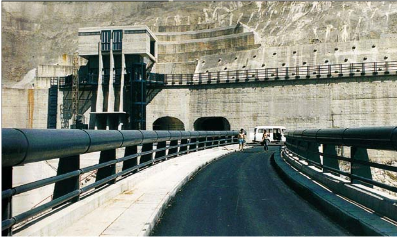
Fig. 53. The guardhouse with the station for operating the outlet valves and for the acquisition and digest of instrument results installed at the ROSAMARINA dam on the San Leonardo River near Palermo, Italy (photo by C. Gambino, 2002)
