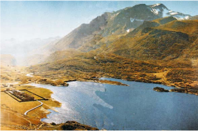
Fig. 106. Views of the territory around the MONCENISIO reservoir on the occasion of a drawdown; a partly destroyed old ospice from the WWI days [44]
